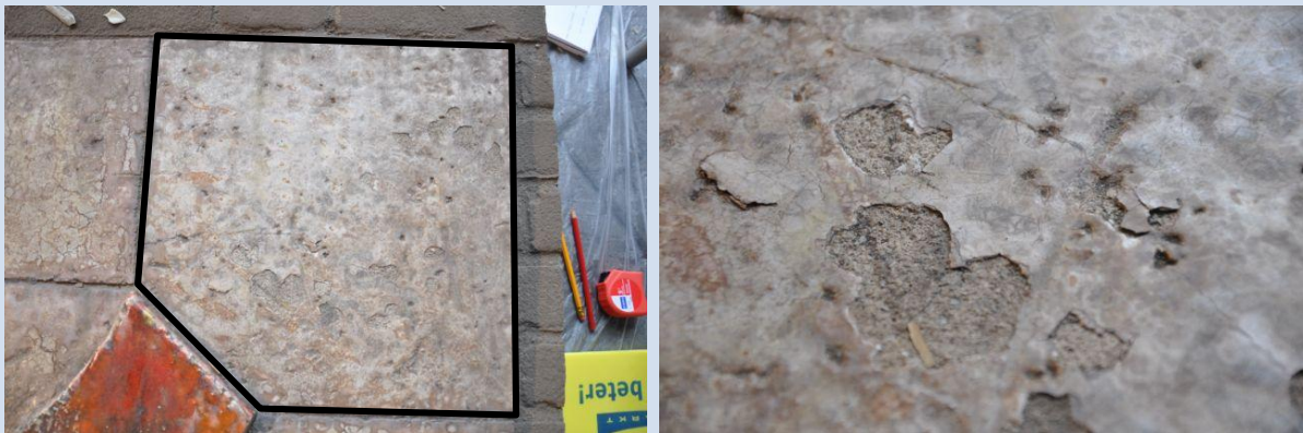
Detail glazuurverlies
