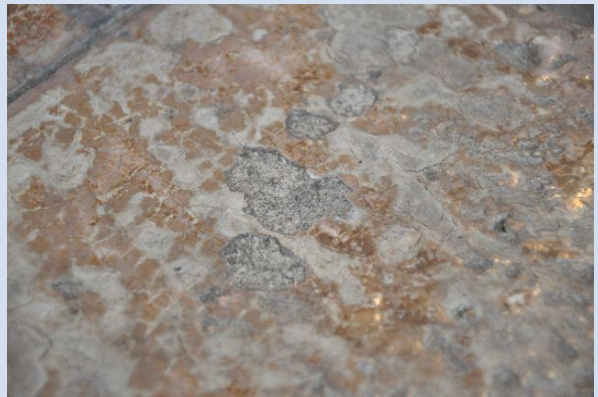
detail glazuurverlies
